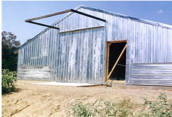
**Building erected using sheets from a bundle of galvanized sheets that had extensive amounts of white rust.**
